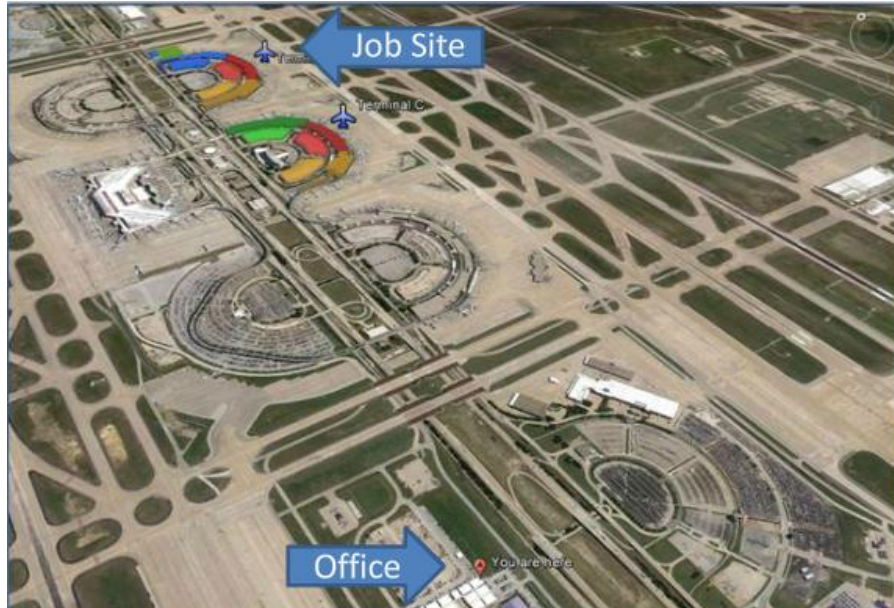
Figure 8.1: DFW Airport Jobsite Aerial View
